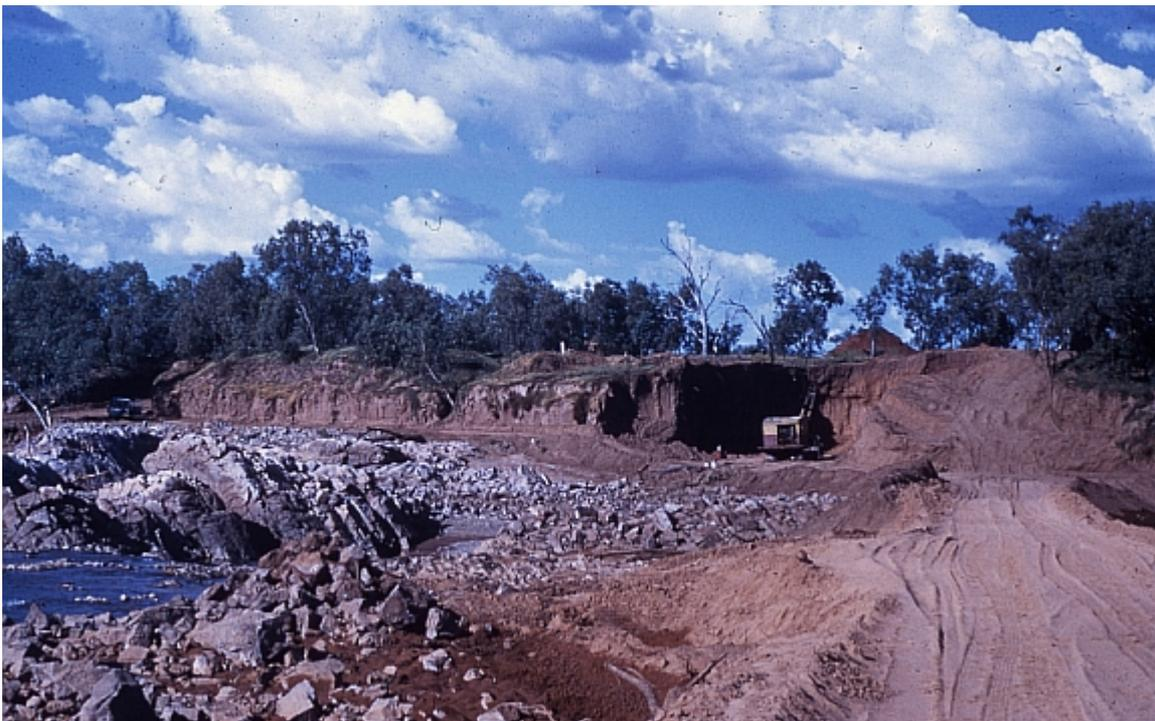
*Excavating for the Diversion Dam east bank abutment (“monolith 47”) - where the roadway approach will be – Circa May 1961. – Unknown photographer*
